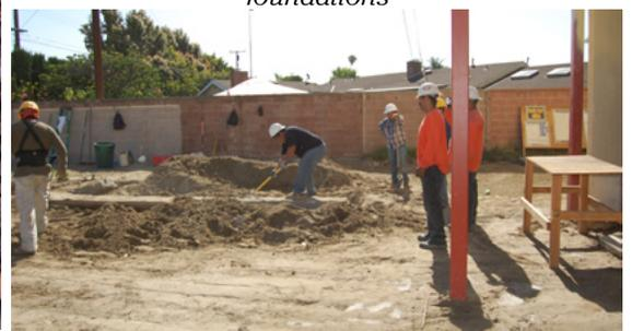
*Using sledgehammers to break concrete footing*
