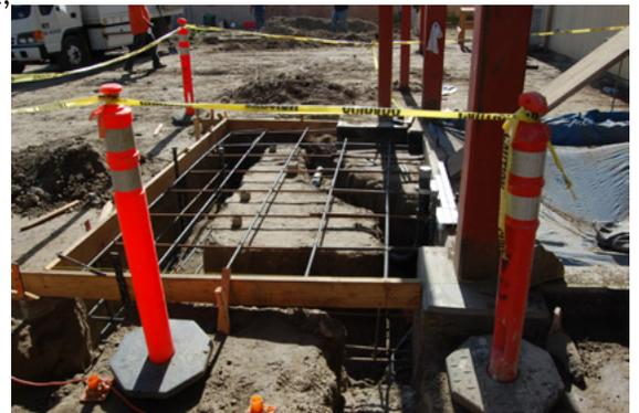
*Elevator mechanical room ready for concrete*
