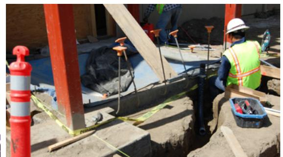
*Electrician installing the conduit pipes in the elevator mechanical room foundations*
